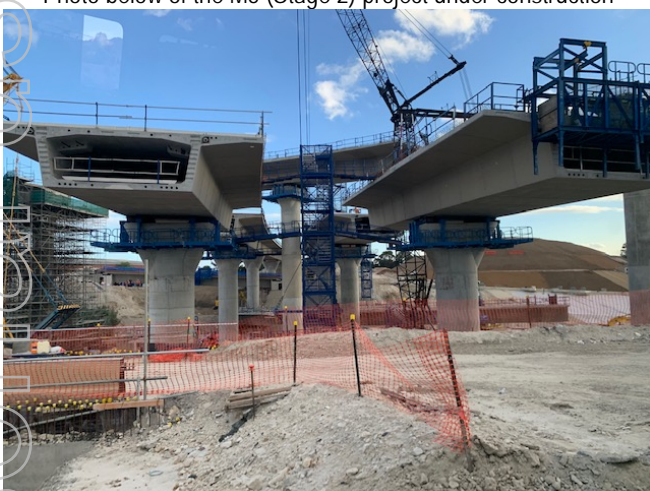
Photo below of the M5 (Stage 2) project under construction
