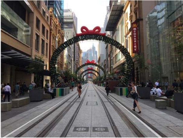
The picture above shows the recently completed light rail section on George Street in Sydney (between Market and King Streets).
